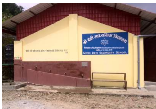
Child-friendly taps set at varying heights to accommodate different ages.
